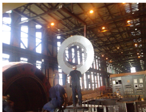
Figure 4. Monolithic end pack of the stator magnetic core in the process of mounting for turbo-generator n. 1 in TPP Bitola
