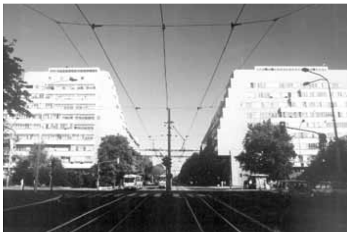
Сл. 15. Н. Добровић, Комплекс ДСНО, 1954-1963. Fig. 15. N. Dobrović, The Complex of DSNO (Total National Defense and Civil Self-Protection), 1954-1963
