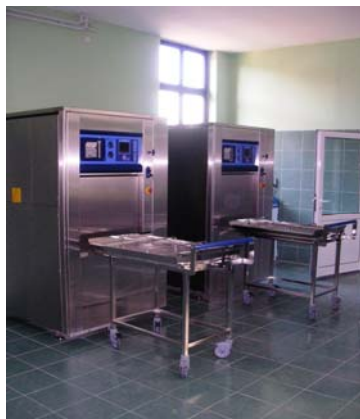
Figure 3 - Autoclaves for the treatment of infectious healthcare waste
