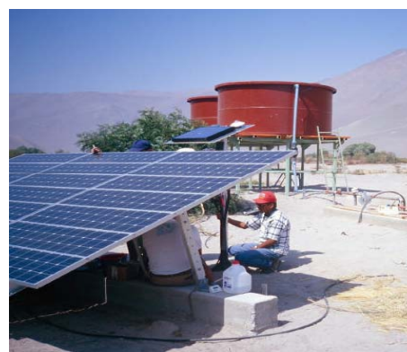
Fig.1. Photovoltaic irrigation system
