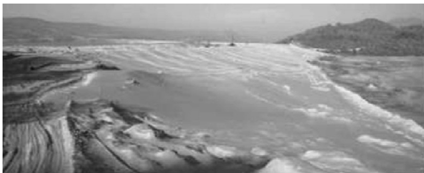
Figure 3 Dam 2 of the Veliki Krivelj flotation tailing dump (2011)
