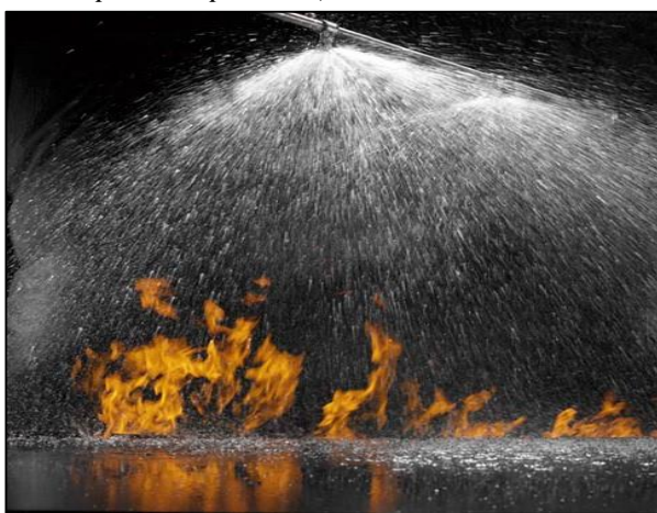
Figure 2 - Sprinkler system in action (figure source: http://allsafefiresprinkler.com/ )
