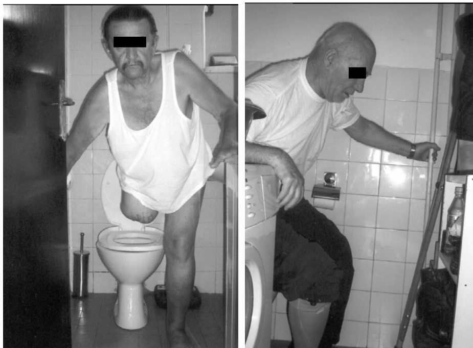
Fig. 1 – Low toilet bowls without adequate supporters
