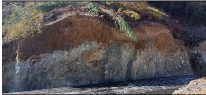
Figure 9 - Terrain cut near the southern portal of the "Crni Vrh" tunnel on Vc Corridor, Bosnia and Herzegovina
