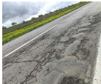
Figure 5 – Slight rutting indicating initial surface deformation
