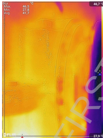
Figure 9 – Thermal image at the gearbox output
