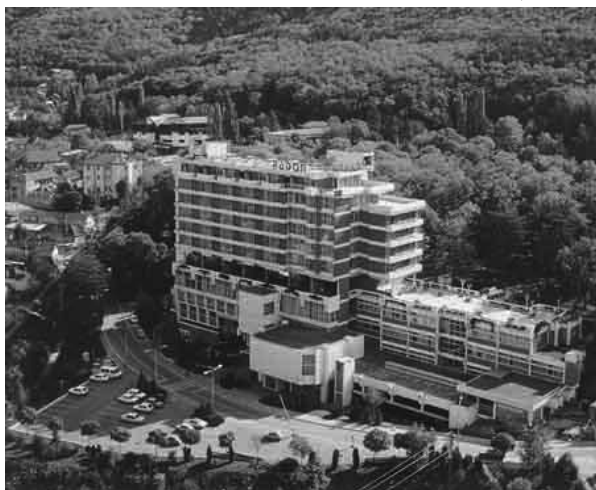
Figure 3. Hotel Radon in Niška Banja, air view (figure source: http://wikimapia.org/11425042/sr/РАДОН ).
