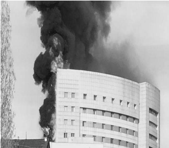
Figure 2. Huge fire in hospital in Istanbul (figure source: https://www.news.com.au/world/middle-east/major-fire-breaks-out-at-hospital-in-istanbul-turkey-patients-evacuated/news-story/0b4efabde0ff457610a5f2b33b2509d0 ).
