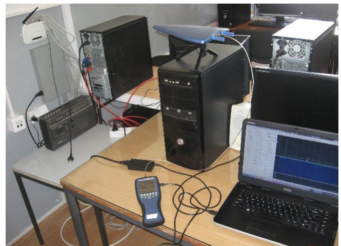
Picture 2d. Routers in different laboratories, TL-WR740N u in laboratory 110
