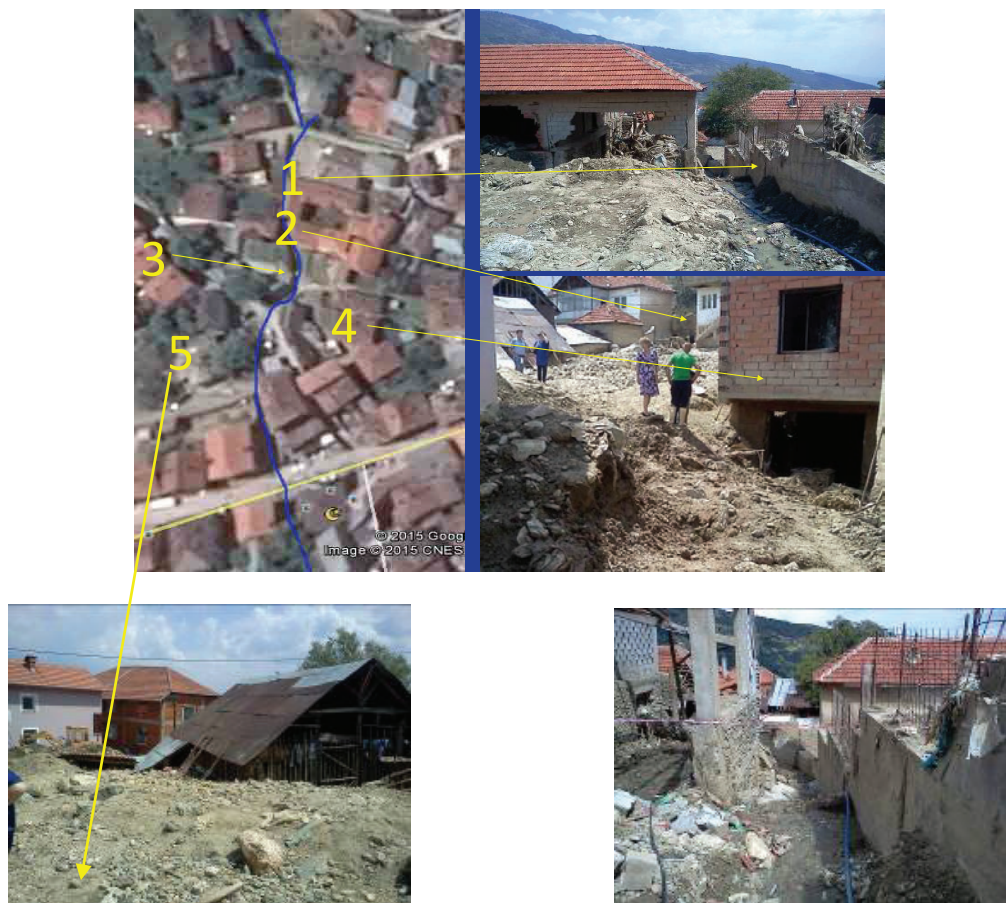
Figure 12. Location of structures along the torrent
