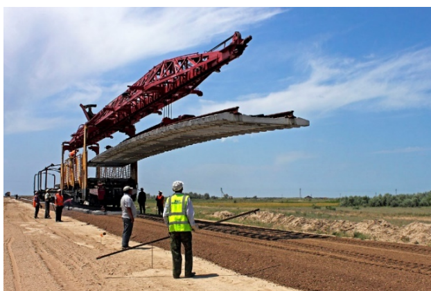
Figure 4 - Crane UK 25-28 for track laying [3] Slika 4 - Kran UK 25-28 za polaganje koloseka [3]
