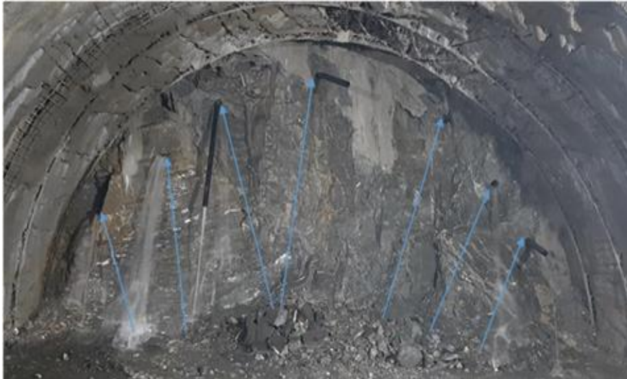
Figure 10. Drainage holes' placement
