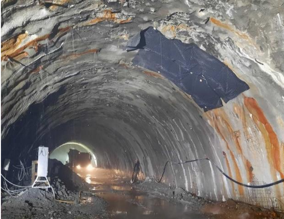
Figure 4. The presence of water in the form of dripping
