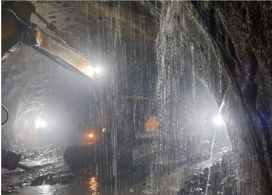
Figure 5. The presence of water in the form of flow
