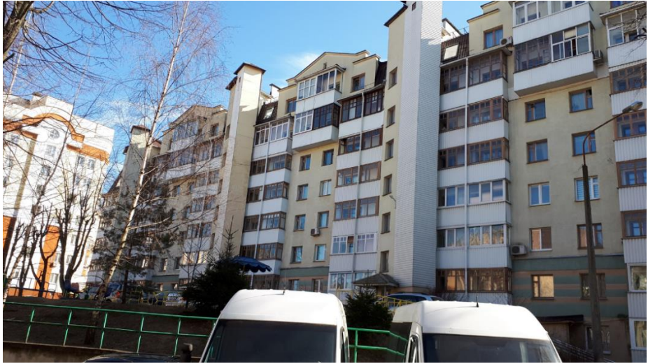
Figure 4 The rear facade of the building with additional external elevators attached.
