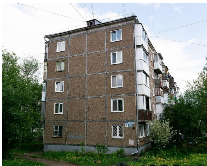
Figure 1 - Typical panel building series 1-464
