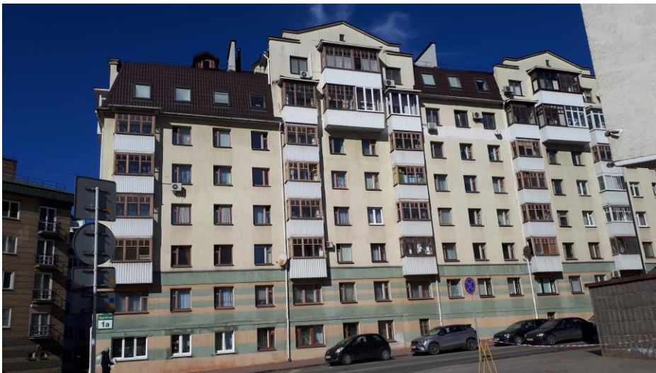
Figure 3 typical series 1-335 after reconstruction
