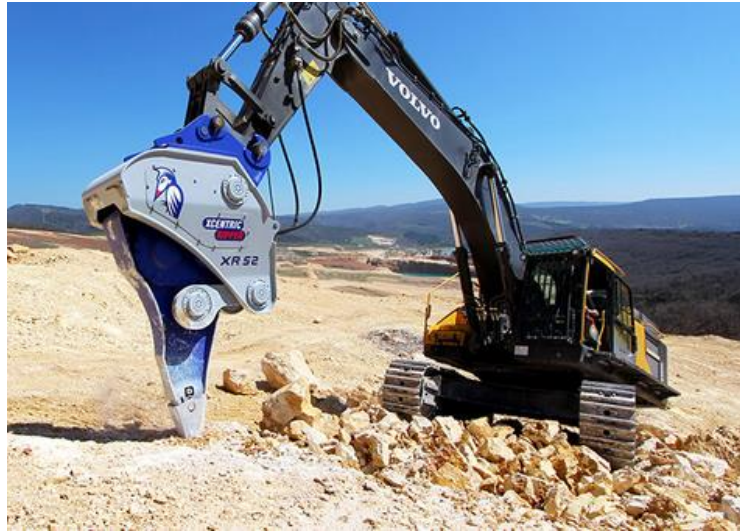
Figure 14 Hydraulic excavator with the ripper (Xcentric, 2023)
