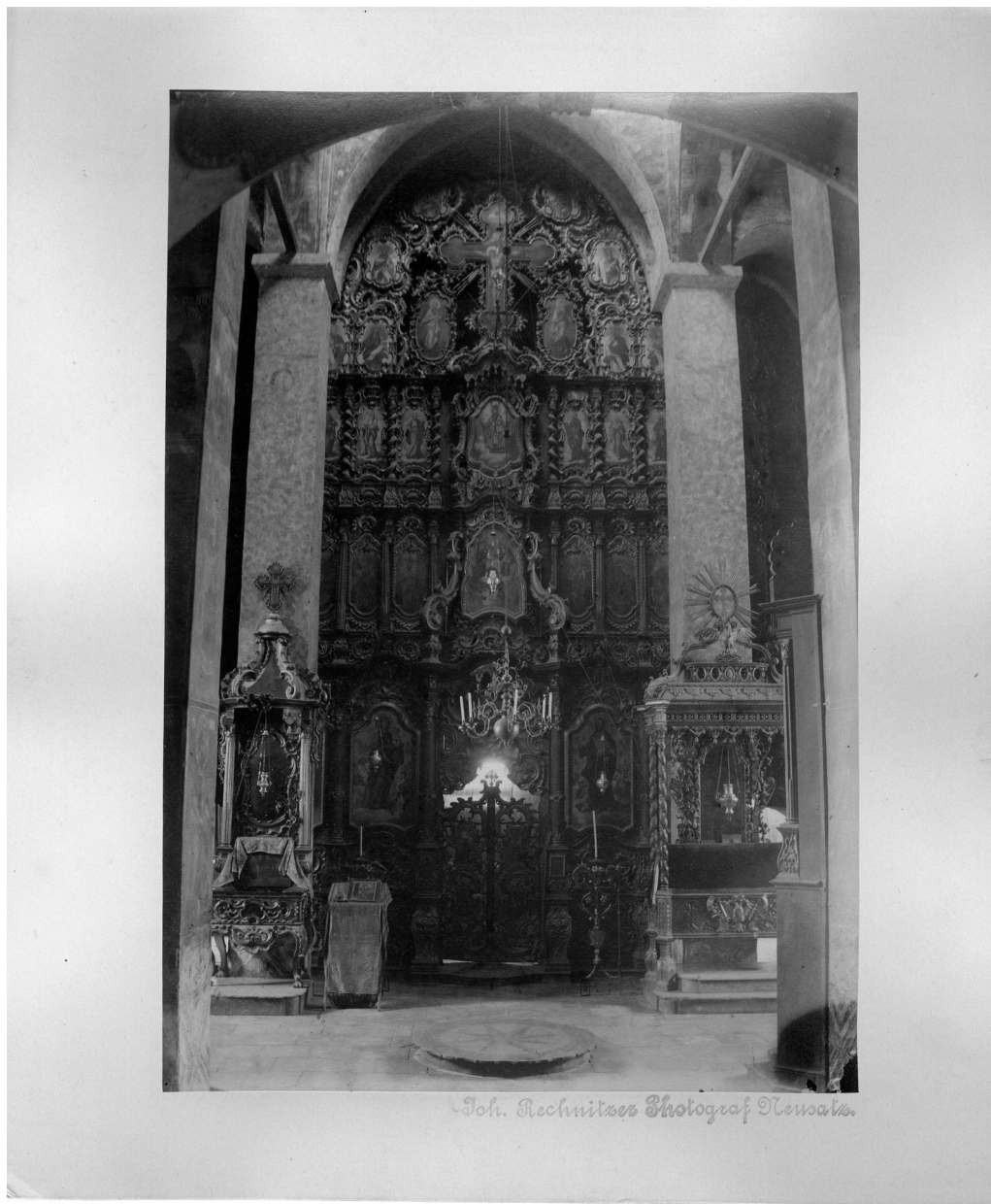
FIGURE 1: EAST SIDE OF THE NAVE IN FRONT OF THE ALTAR, SASA ARCHIVES, 14484; 70533/11, BOXES XXXV.
