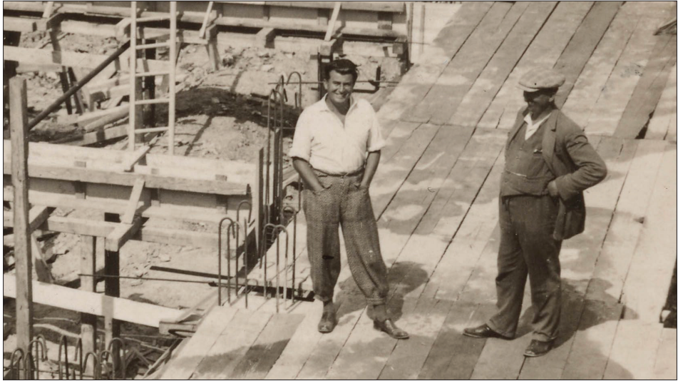
Figure 3. Nikola Dobrović with a worker at the construction site of the Grand Hotel, Lopud near Dubrovnik, 1936. The Museum of Science and Technology, Belgrade.
