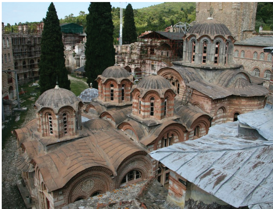
Fig. 1. Hilandar Monastery, katholikon viewed from southwest; from right to left: domed naos, twin-domed inner narthex, and single-domed exonarthex (photograph by author).
