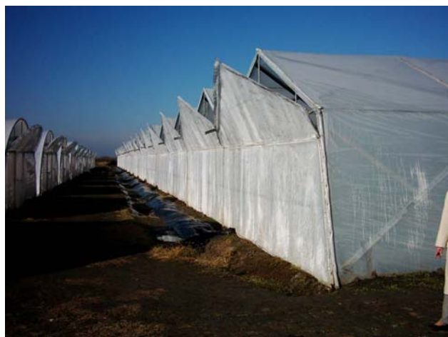
Sl. 7. Sistem provetravanja Fig. 7. Ventilation system
