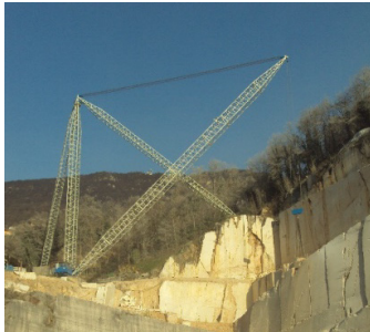
Figure 1 Derrick crane used in this research.
