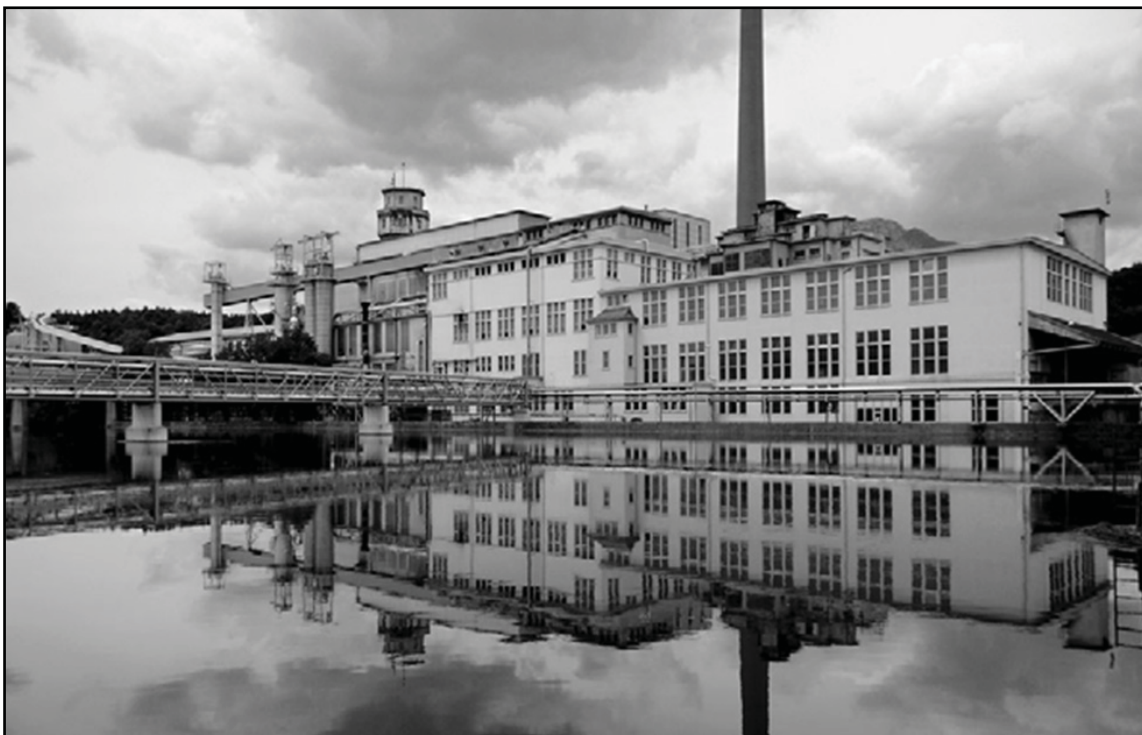
Figure 1: Ex-wood-industry complex in Solothurn, Switzerland
