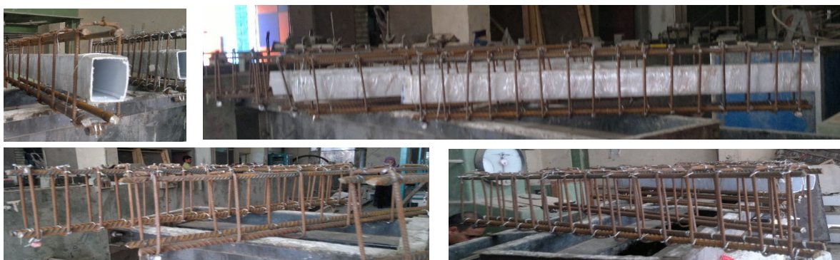
Fig. 2. Steel Reinforcement Bars and Plastic Box [4]
