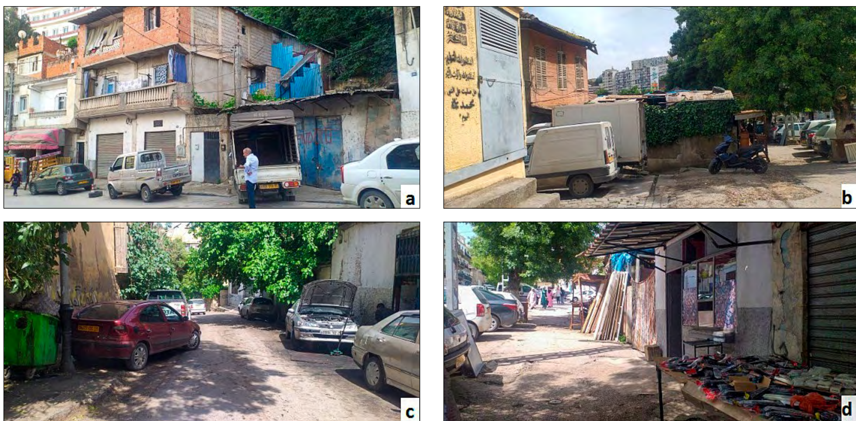
Figure 5. Condition of Avenue Rahmani Achour
