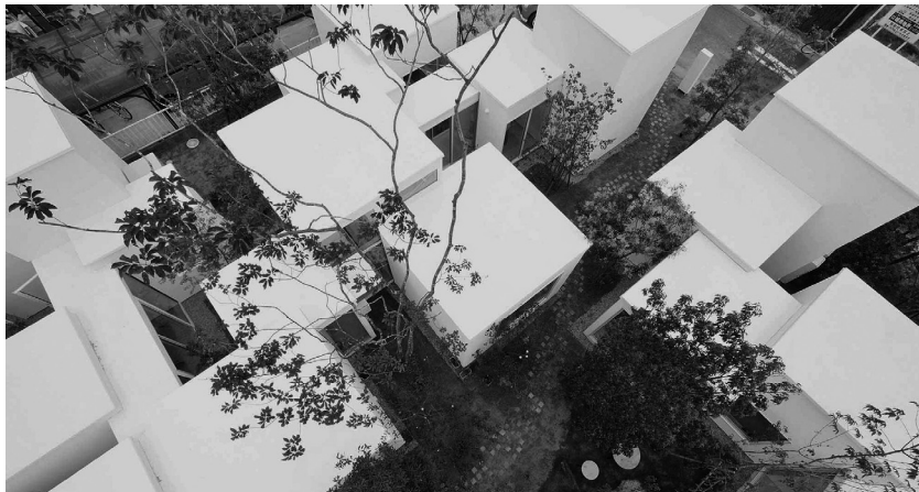
UP: FIGURE 7: Row of Houses 28
