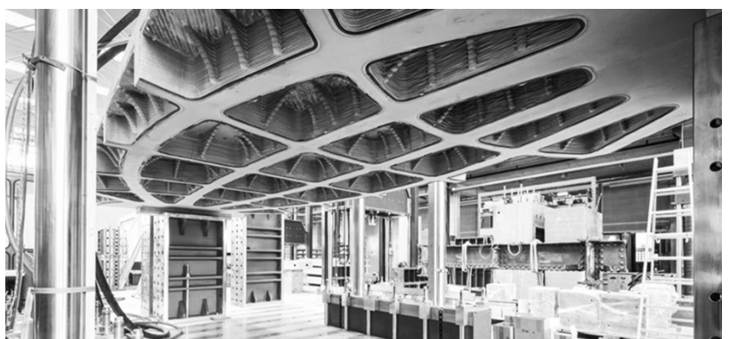
FIGURE 10 COEBRO Ribbed Slab, Hansemann, Georg, Robert Schmidt, Holzinger Christoph, and Joshua Tapley. "Additive Fabrication of Concrete Elements by Robots: Lightweight Concrete Ceiling." In Fabricate 2020, 124–29. UCL Press, 129, figure 8
