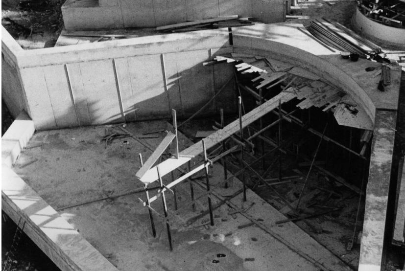
FIGURE 8: Photograph of the construction site by Giacomo Calò Company
