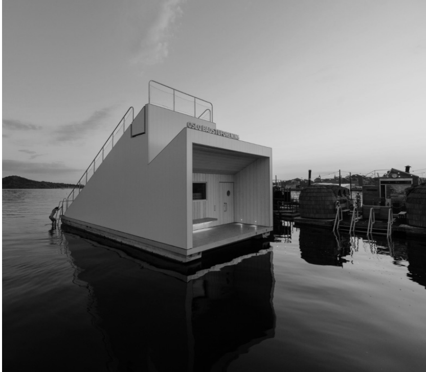
FIGURE 2a. Trosten Sauna - floating unit in a semi-natural fjordcontext.
