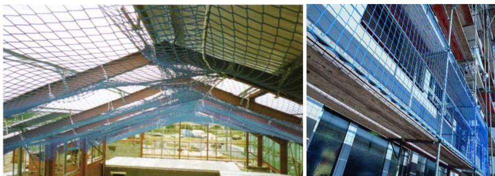
**Figure 3.** Fall arrest safety net [7-11]
