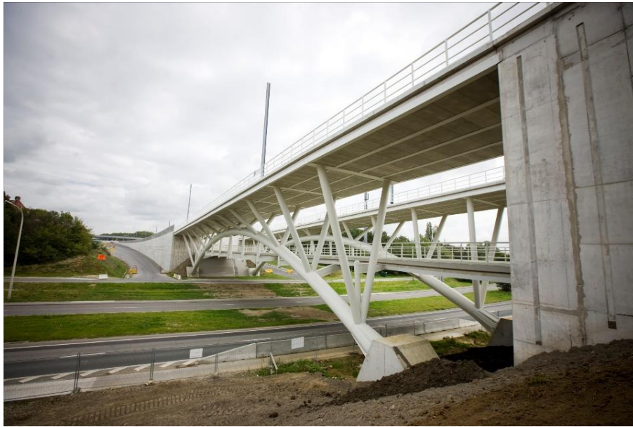
Figure 2. Woluwe Lane Bridge
