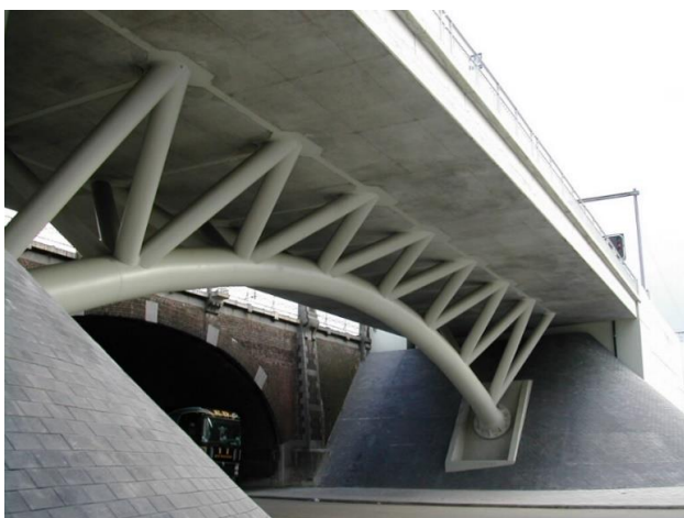
Figure 1. Merxem street tubular arch bridge
