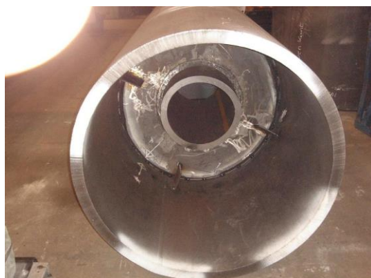
Figure 8. Fabrication of internal stiffening
