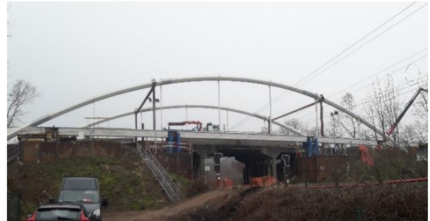
Figure 22. Bridge with temporary bracing
