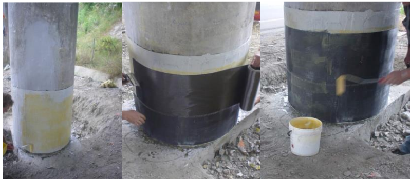
Figure 4.3. Confinement strengthening (Di Ludovico M. [21])
