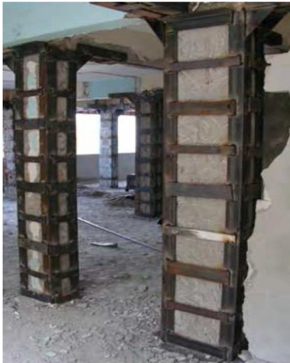
Fig.2.5. Steel jacketing applied to RC columns(M.N.Fardis, [12])
