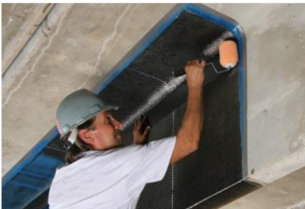
Figure 4.4. FRP strengthening of a beam (CNR-DT, [8])
