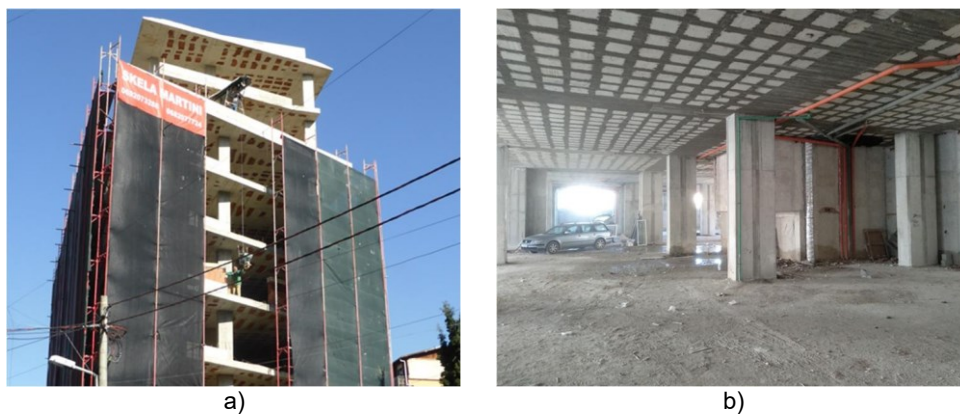
Figure 2. Typical examples of RC frame buildings in Albania: a) a building during construction, b) interior of an existing building
