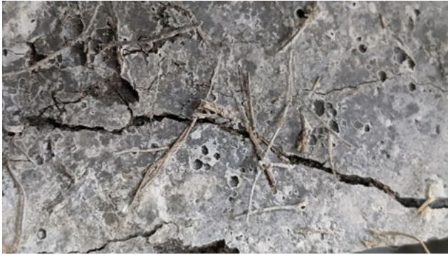
Figure 14. Failure pattern of fiber reinforced beam specimen
