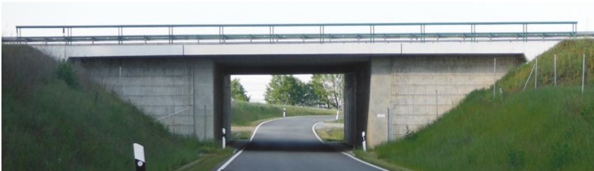
Figure 6. Single-span concrete slab bridge
