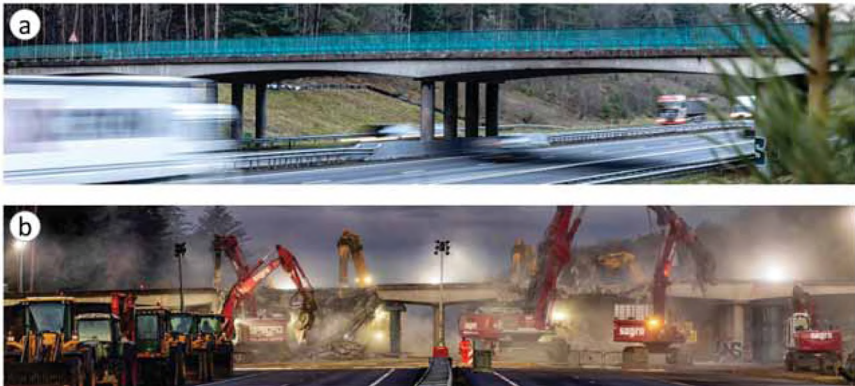
Fig. 1. Demolition of Hoog Burel viaduct (A1), the Netherlands: a) before demolition, b) during demolition (November 2022). Credits go to Rijkswaterstaat [10]
