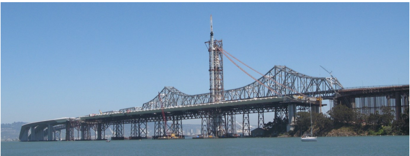
Figure 13. New East Bay Bridge under construction (2011)
