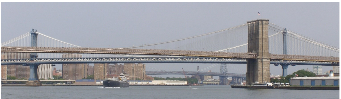
Figure 9. Brooklyn, Manhattan and Williamsburg Bridges across East River, New York City
