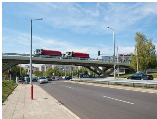
c) Steel road bridge
