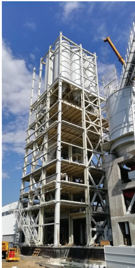
a) High-rise industrial steel structure with CBFs
