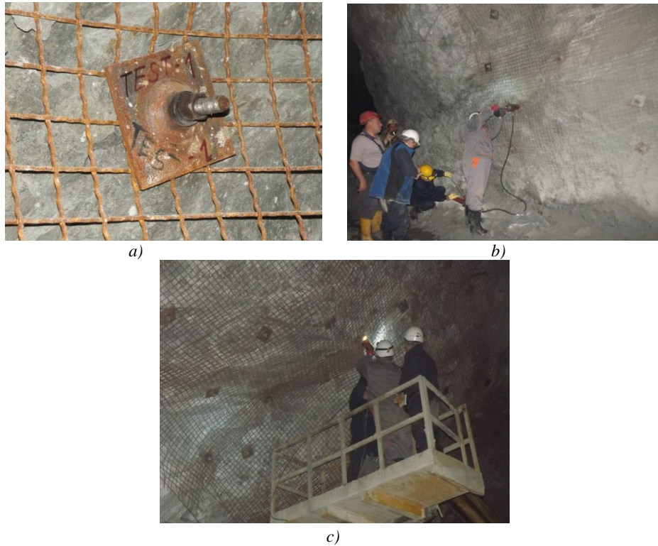
Figure 1.1 a), b) and c) Testing of anchors - determining the pull-out force
