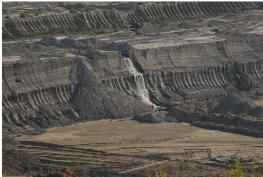
Figure 3 The open pit "Drmno" after the instabilities in the slopes
