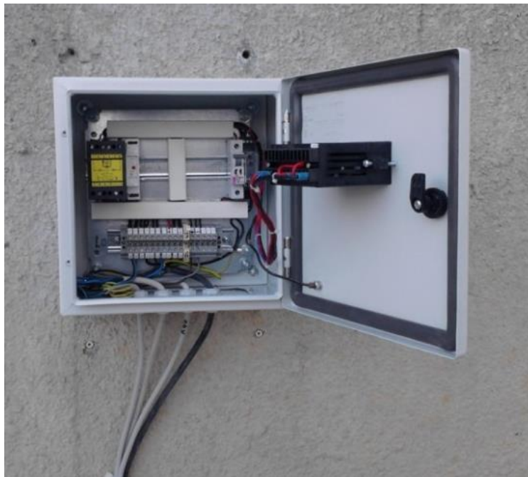
Figure 6 Transducer applied for the electric motor overload protection [8]
