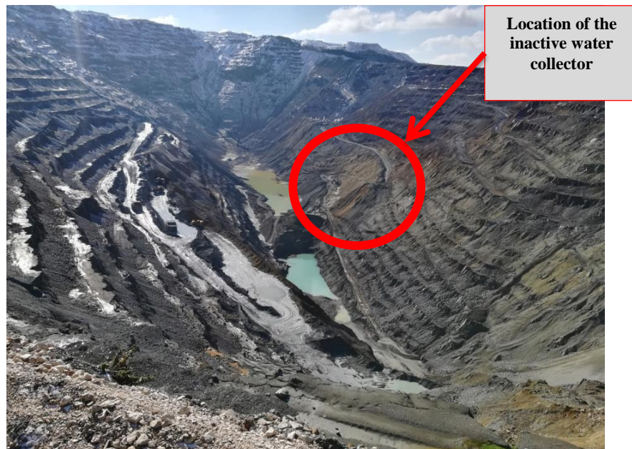
Figure 1 Location of the water collector at the level L+150 m on the bottom of the South Mining District Majdanpek Mine (north side view)
