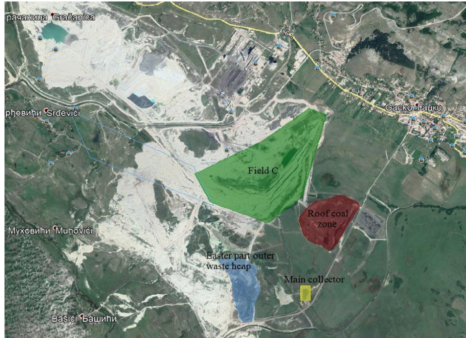
Figure 1 Layout of the mining facilities at the open pit Gacko
