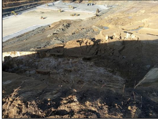
Figure 1.1 View of the landslide from the above (December 2020)
