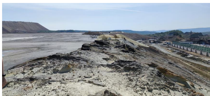
Figure 2 Detail of the endangered part of the embankment between PPS and Dam II, flotation tailing dump RTH, 2021
