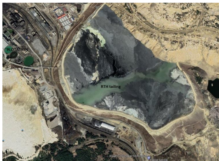
Figure 1 Flotation tailing dump RTH, GoogleEarth source, taken on April 9, 2021
