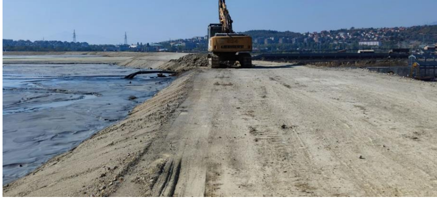
Figure 5 Embankment between the Dam 2 and high landfill, October 5, 2021
