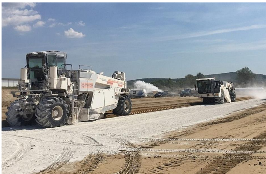
Figure 3 The process of stabilizing the base soil with lime in the field [2]
