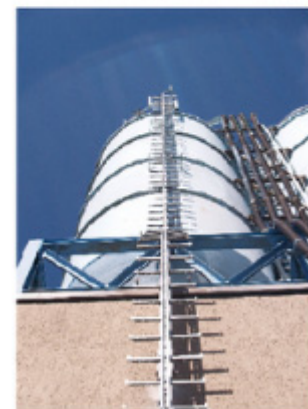
Figure 2: Example of construction of guided-type fall arrester with rigid anchor line made of rail (Vertiqal Engineering production) [13]
