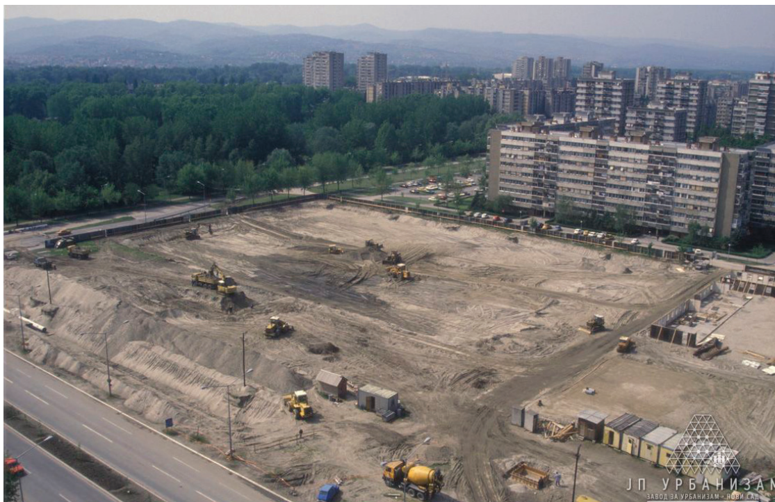
Fig. 2. Appearance of the formed Liman and preparations for the construction of the „Nafta-gas“ building at the intersection of the People's Front and Liberation Boulevard (Source: URBIS).
